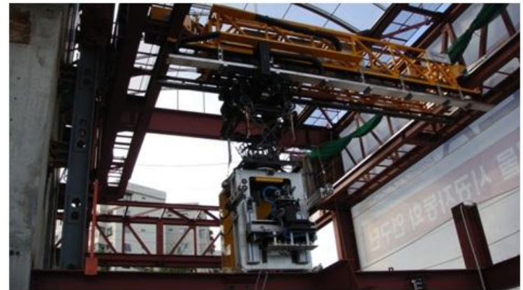
Fig. 5. Integration of robotic automation system for steel beam assembly
