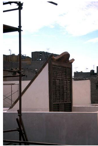
Fig. 3. The Malqaf of the Main Palast Zisa, Sicily, Qa-a of the Suheimi House [13]
